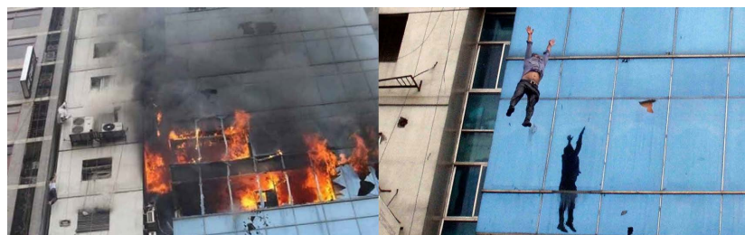
Figure 1. FR Tower Fire hazard at Banani (source: Monirul Alam, Apurbo Chowdhury).
