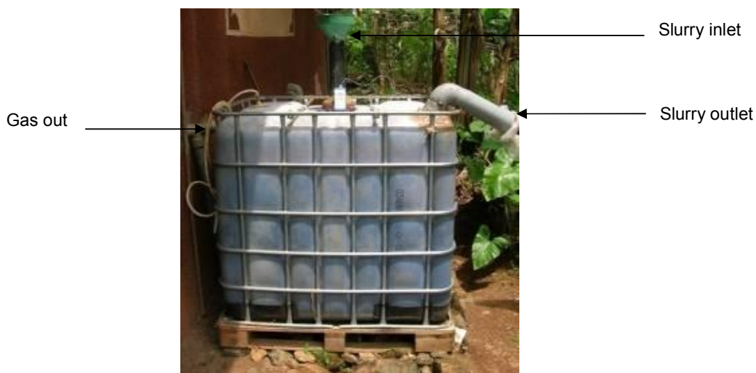
Fig. 1. A 1000l biogas digester for cowdung
